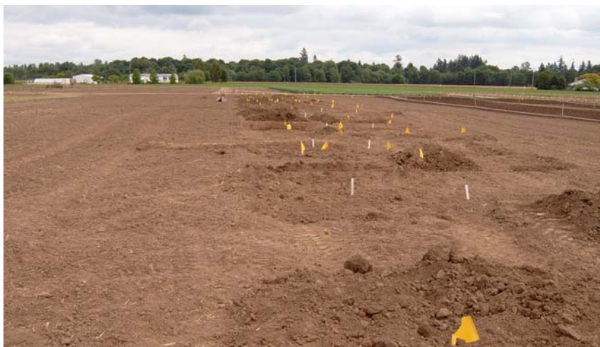
Site after pits were dug
