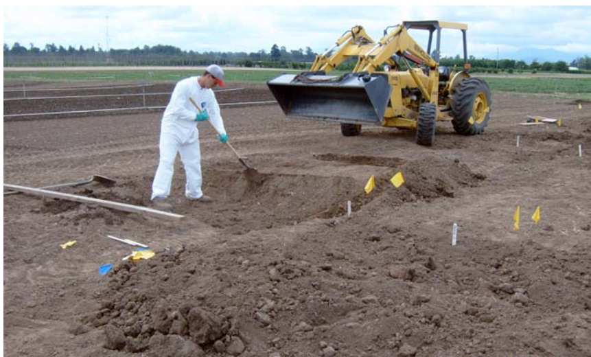
Preparing pits for application of fumigant.
