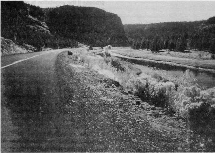
Photo 1. The Crooked River in central Oregon. There is nothing crooked about this stretch, which was straightened during road building. (Photo courtesy of John Buckhouse).
